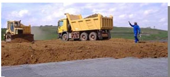
Topsoil cover being end tipped on top of the cell to anchor the slopes
