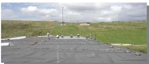
The Secugrid® being positioned prior to topsoil covering
