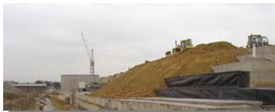
The primary clay capping layer being placed to shape the cell
