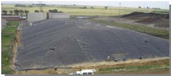
The 1,5 HDPE liner installed over the cell
