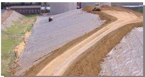
Top of the cells had to be completed before the side slopes could be covered.
