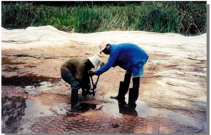
Fixing panels of *Flexmesh* over the wetland. Note wire mesh and transverse steel rods over the geotextile.
