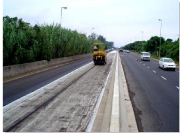
Rehabilitation under construction. KayTech's Sealgrid™ is installed prior to the asphaltting.
