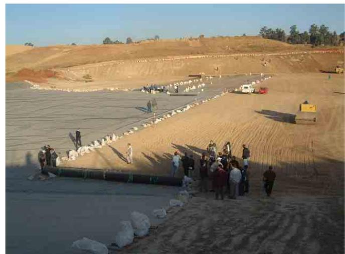
**Photo 3: Installation of HDPE geomembrane liner**
