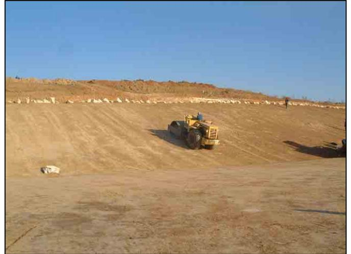
**Photo 2: Compaction of the clay layer**
