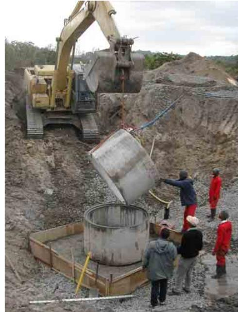
**Figure 2:** Construction of subsurface drainage pump station for leachate pond
