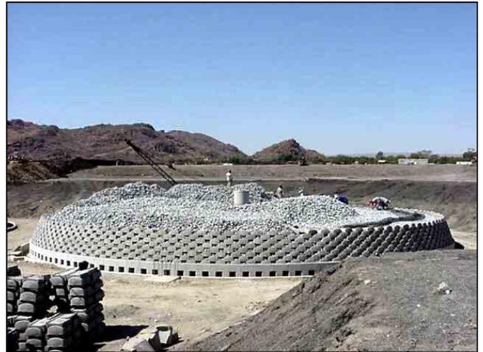
Photo 1: View of the Mothutlung biofilter
