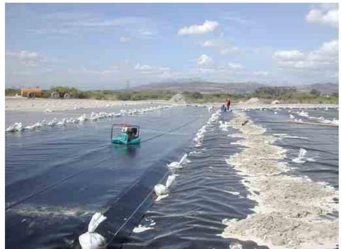
**Figure 3:** LLDPE liner at central drain of Cell 1
