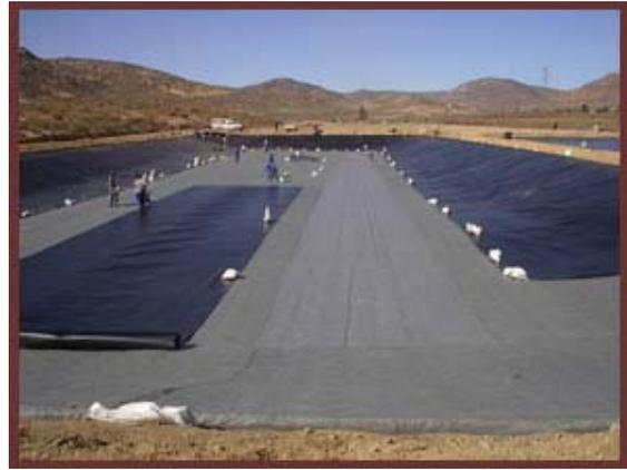
A 240 g/m<sup>2</sup> geotextile was used as a liner protection layer
