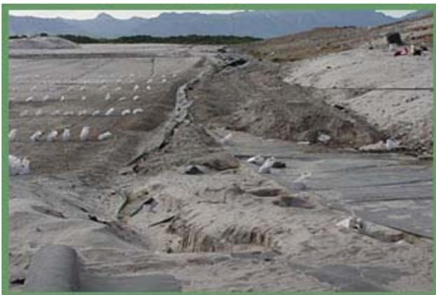
Figure 2 - Connecting the new lining system to the existing liner
