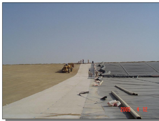
Bentofix GCL and Carbofol HDPE liner being installed
