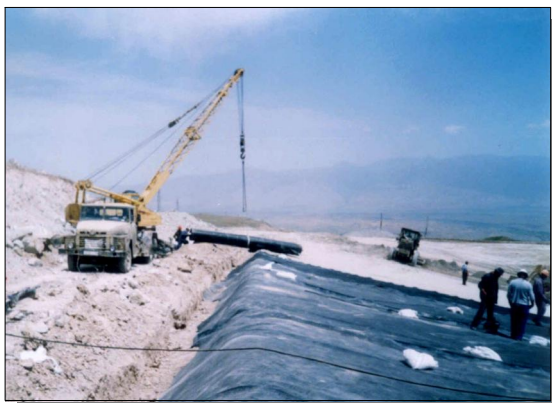
Picture of cable operated crane used to move material on site
