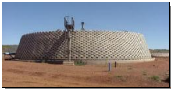
The placing of the stone at the Delmas project.
