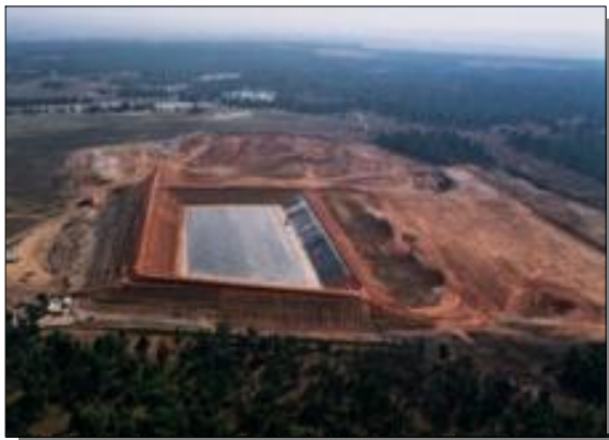
Aerial view of site during construction
