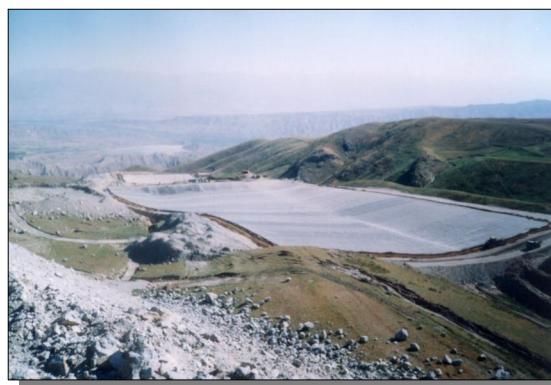
A view of the pads in the hilly terrain of Tajikistan
